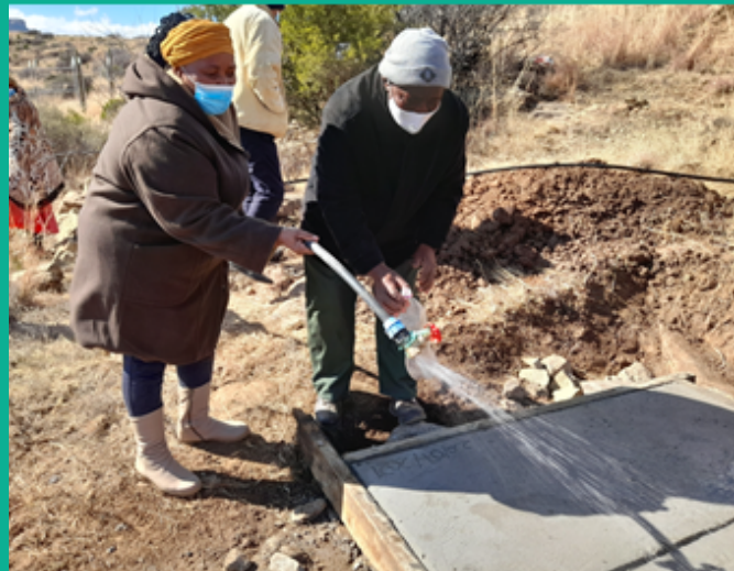
Project members testing the water supply
